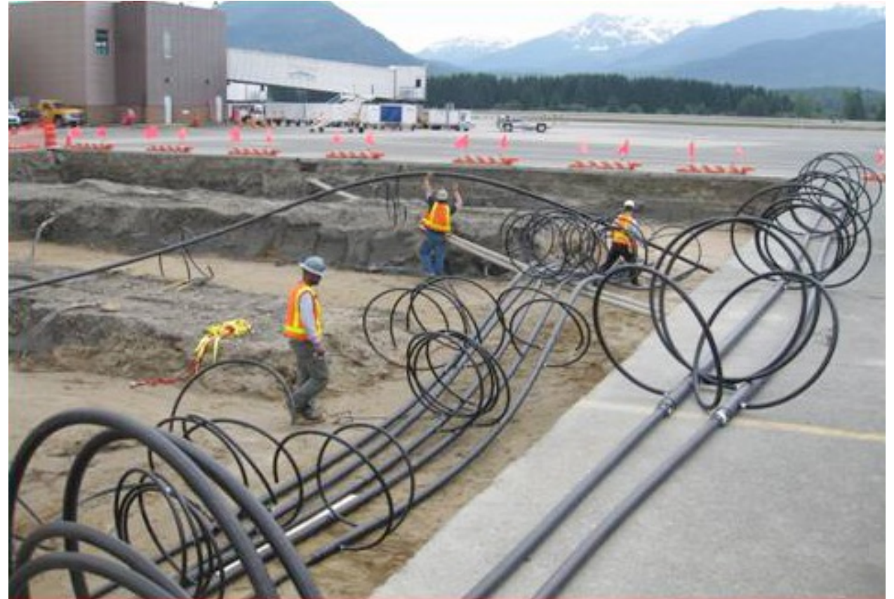
Installation work on the ground source heat pump loop for Juneau airport, 2012
