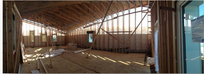
Buckland prototype house under construction.
