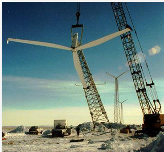
Kotzebue Electric Association wind turbine being raised. Photo courtesy of KEA.
